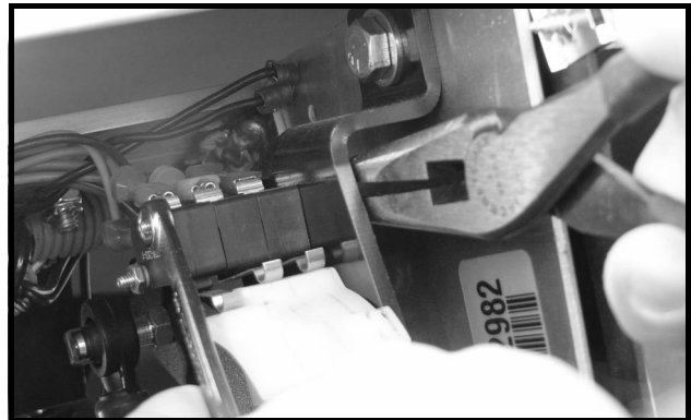
Figure 14-19 Removal of Limit Switches
